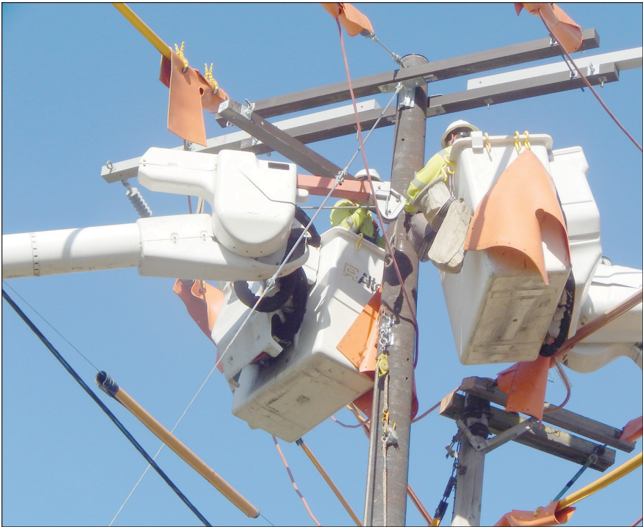
▲ PHOTO | TRI COUNTY Joe Monroe, foreman, and Wesley Meador, supervisor, with Groves Electrical Service, finish tying into intersecting electric power lines from the former existing transmission lines (right) to the new lines (left) without interruption of electricity to households and businesses. Lineman received training with four months of lineman school and four years of apprenticeship.
