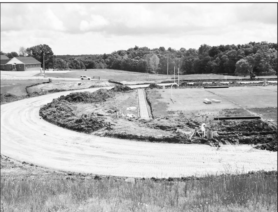
WORK CONTINUES AT Trojans Field where a number of contractors are removing the old track and replacing it with an oval that will allow the local high school to host track meets. A new drainage system is also being installed along with a watering system for the football field and new lighting at the facility. Work is expected to be completed in time for the fall sports season.
